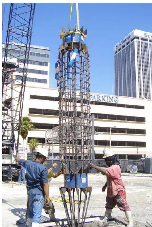
Assembly of a multi-level O-cell arrangement
