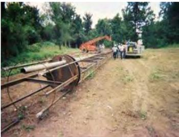
1 of 8 O-cell tests ready for placement
